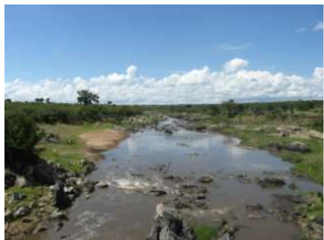
New Mara Bridge – December 13 th , 2009
