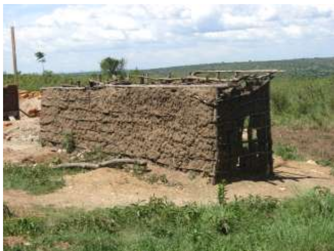
Picture 6: Latrine currently in use at the Mbalibali Primary School.
