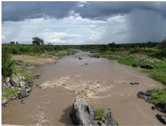
New Mara Bridge – May 15 th , 2009
