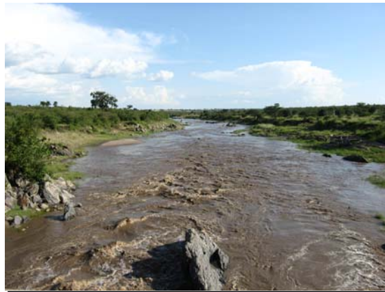
New Mara Bridge – June 1st, 2009
