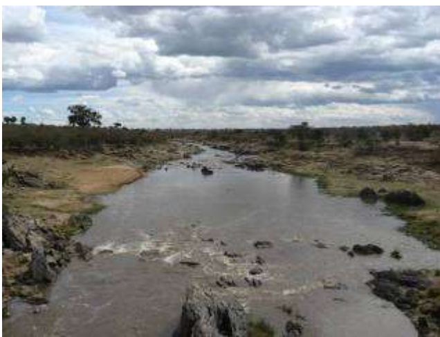
New Mara Bridge – October 15 th , 2009
