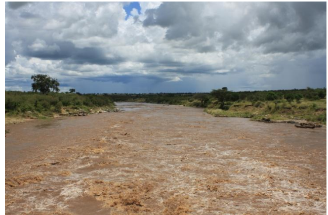
New Mara Bridge – April 3 rd , 2010
