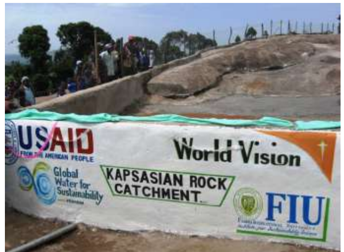
Picture 2: Commissioning of the Kapsasian Rock Catchment
