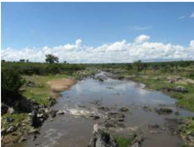
New Mara Bridge – December 13 th , 2009
