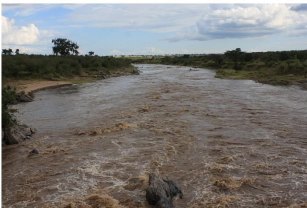
New Mara Bridge – May 16 th , 2010
