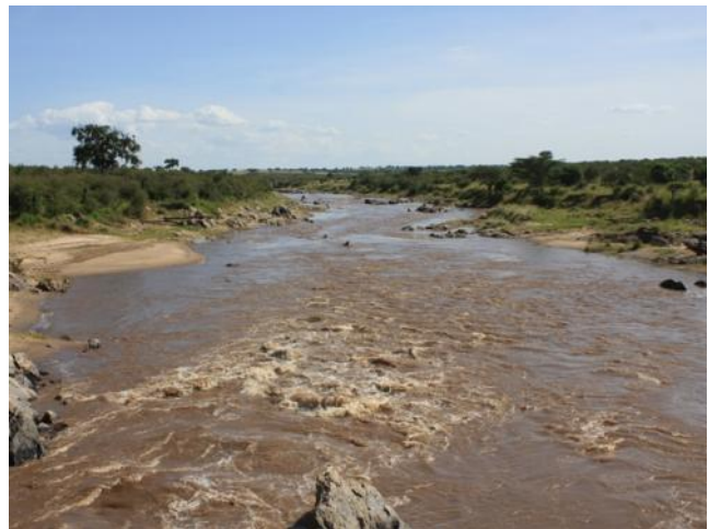
New Mara Bridge – March 14 th , 2010
