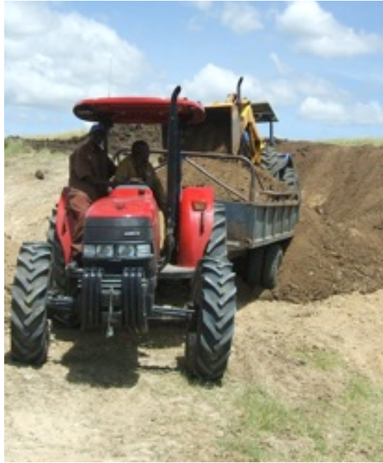
Road Team collect murrum to repair roads.
