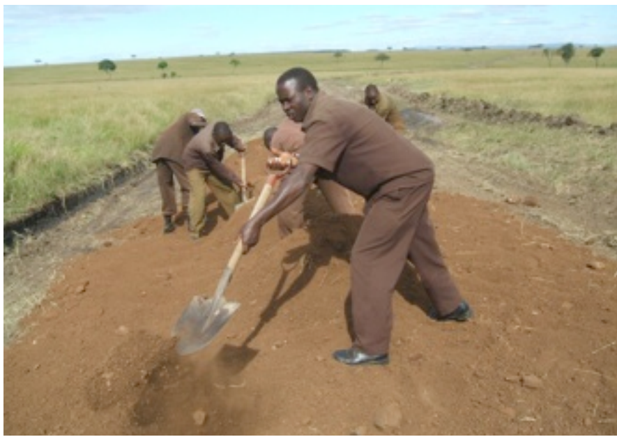
Road Team patching up the main road. Taken by Simon Matara.
